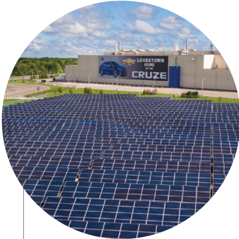
GM solar installation; Lordstown, OH.
